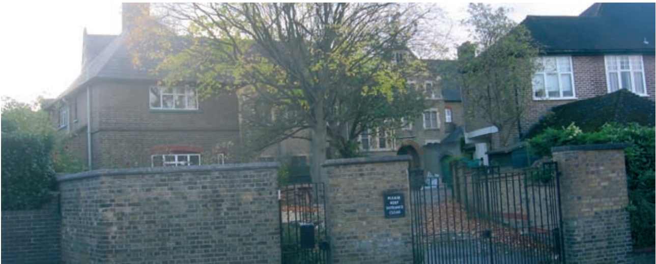
Main entrance on Bridge Lane
