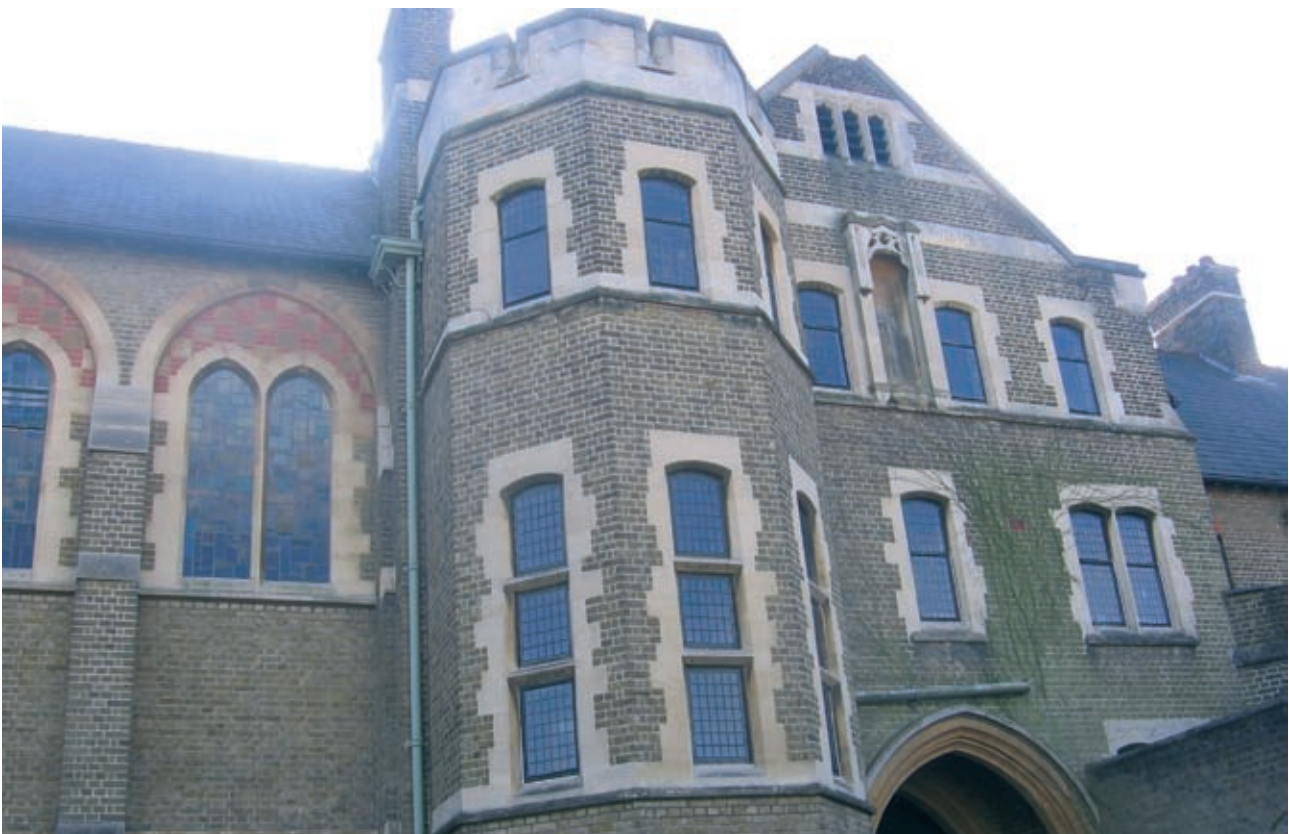
North, front elevation of the monastery
